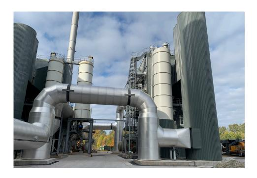
Because of regulatory requirements in summer 2006 Interprojekt added a SCR reactor with catalysts and ammonia water storing and dosing system to the existing installation.
